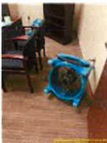
Main Level > Office - B102 > EQUIPMENT [BEFORE] Office - B102 [ Main_Level.Office_- _B102_230620110005.jpg ]
