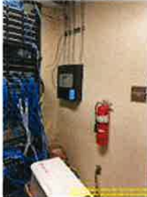
Main Level > Electrical - B111 > BEFORE
