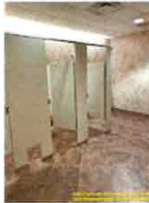
Main Level > Mens > BEFORE
