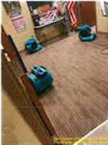
Main Level &gt; VA Waiting - 101 &gt; EQUIPMENT
