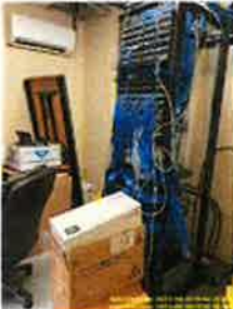
Main Level > Electrical - B111 > BEFORE
