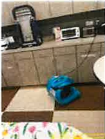
[EQUIPMENT] Work/Break Room -B110 [ Main_Level.Work/Break_Room_-B110_230620145038.jpg ]
