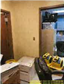
Main Level > Electrical - B111 > BEFORE
