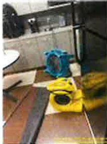
[EQUIPMENT] Work/Break Room -B110 [ Main_Level.Work/Break_Room_-B110_230620145035.jpg ]
