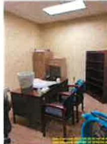
Main Level > Office - B102 > BEFORE [EQUIPMENT] Office - B102 [ Main_Level.Office_- _B102_230620135424.jpg ]
