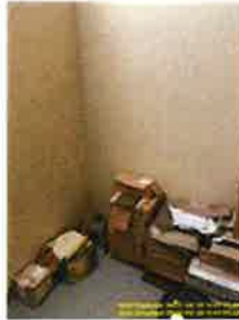
Main Level > Mechanical - B112 > BEFORE
