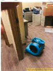
Main Level > Reception- B100 > EQUIPMENT
