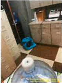
[EQUIPMENT] Work/Break Room -B110 [ Main_Level.Work/Break_Room_-B110_230620145039.jpg ]
