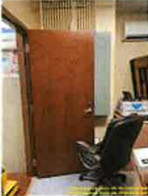
Main Level > Electrical - B111 > BEFORE
