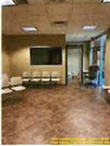
Main Level > Justice Court Lobby > BEFORE
