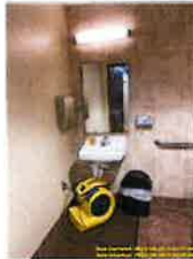
Main Level > Bathroom 1 > BEFORE
