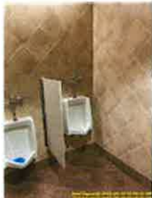
Main Level > Source of loss
